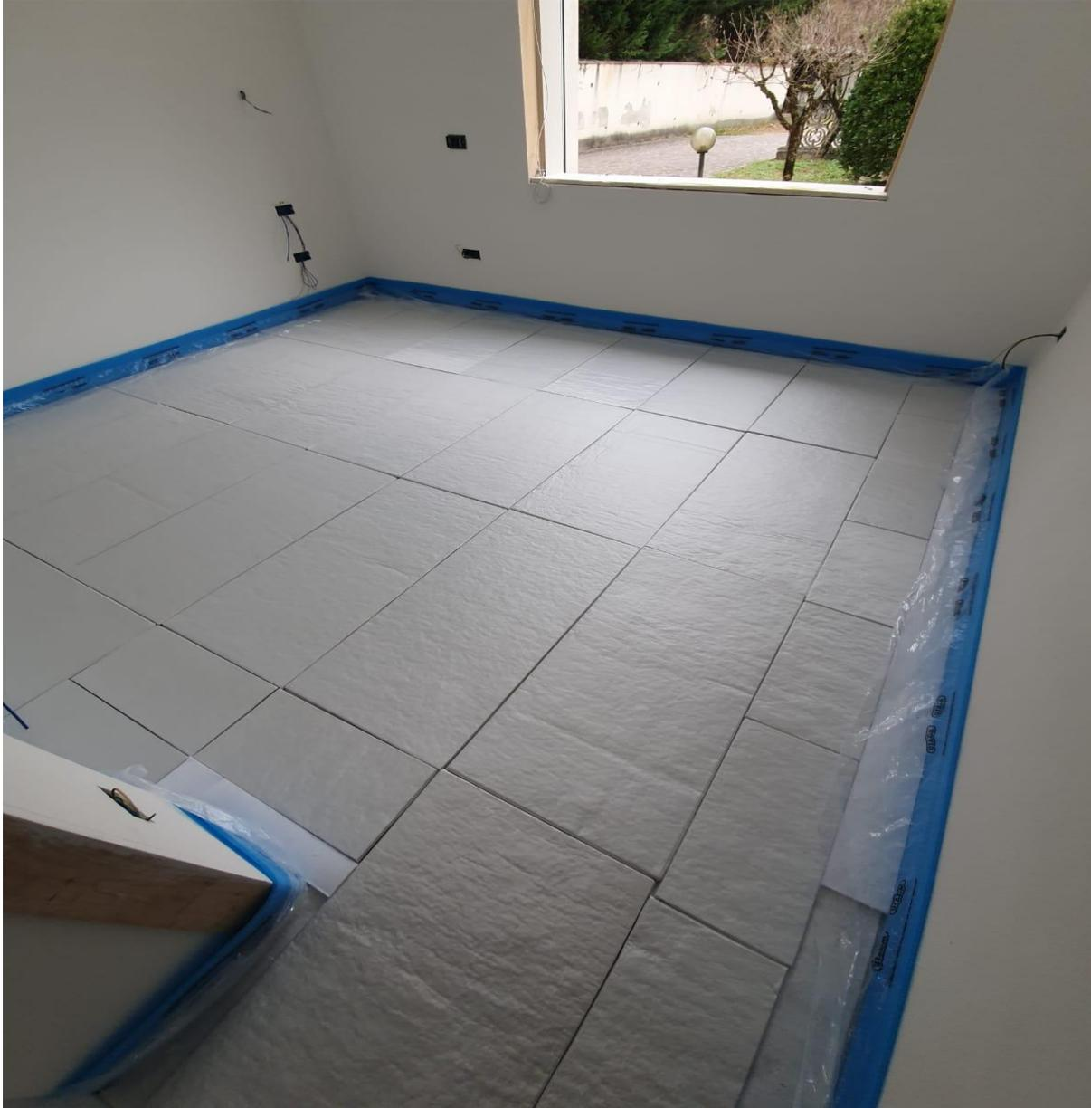
**Note:** It is recommended to tape the joints of the CZ panels and the perimeter of the flooring using an aluminum and bitumen adhesive tape.
