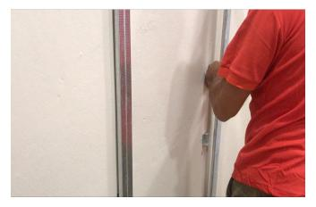
After this stage, the ISOLCORE 'C' posts snap-in need to be installed at an inter axle spacing of 60 cm. This measure can change depending on determined static stanstards, on the fire certificate, on the acoustic, on the impact strength ). If the ceramic cladding is required the inter axle spacing between the struts must not exceed 40 cm.
