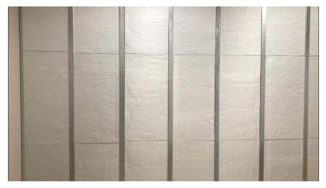
Caution: it is recommended to exercise a light pressure between panel and panel to avoid any joints. It is possible to seal the joints by taping them with ISOL-TAPE silver adhesive, the "American" one.
