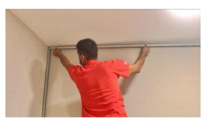
Firstly, attach the top rail to the ceiling, with the right fixings for the support, and place a maximum spacing of 50 cm.
