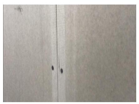
After the drying process has been completed, verify that there are no imperfections along the grouted joint; for this purpose, the spatula over the joint which is placed transverse to the axis, and remove any roughness with the same squeegee or with a fine-grit sandpaper pad.
