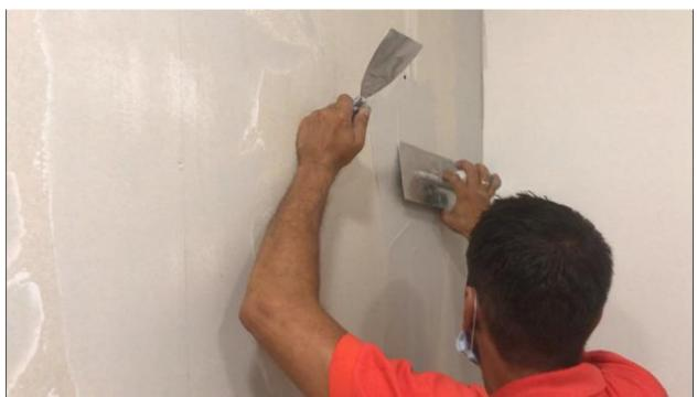
Secondly, apply the second coat of grout, which will extend over a width of approximately 30 cm which is necessary to bring the grouted surface to the same level of the cardboard surface. Next is
