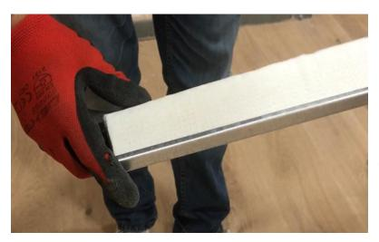
**Note:** In case of depth problems where it is not possible to place the 3 cm CZ panel it is possible, in case the wall is vertical and the height does not exceed 3 meters, to install the structure without the clamps reaching at a total thickness of approximately 2.6 cm
