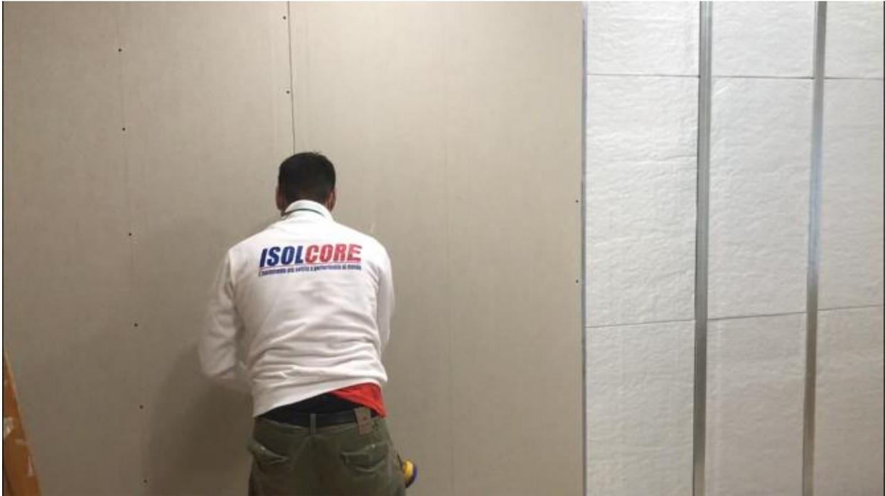
Adjust the tip of the screwdriver so that the nails are at the correct depth, with the top perfectly aligned with the cover of the slab. The nails must be placed approx. 1 cm from the longitudinal edge of the slab and approx. 1.5 cm from the leading edge.
